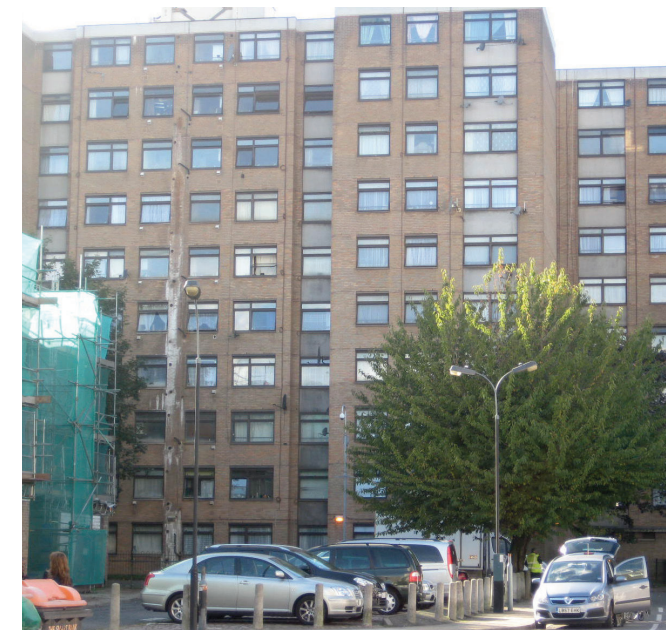
Figure 2.23: Photograph of a housing block within the West Kensington Estate
