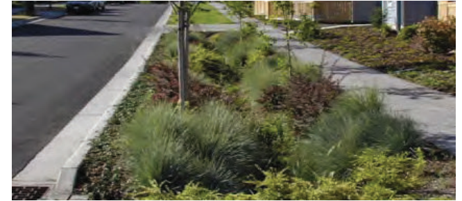
Figure 12.2: Photograph of landscaped drainage channels
