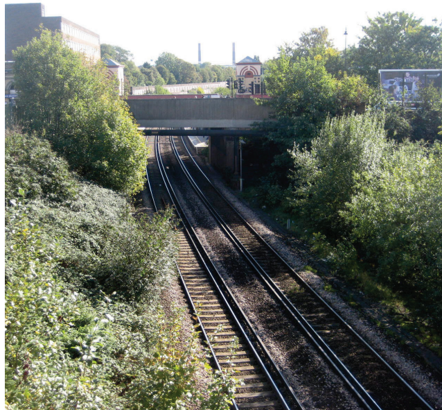
Figure 4.7: The railway line, looking south from EC2
