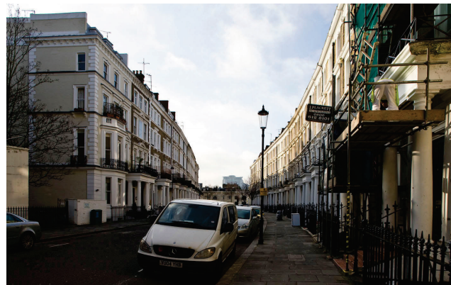
Figures 4.16 to 4.18 (right): Examples of the current impact of the Empress State building on important views towards the OA
