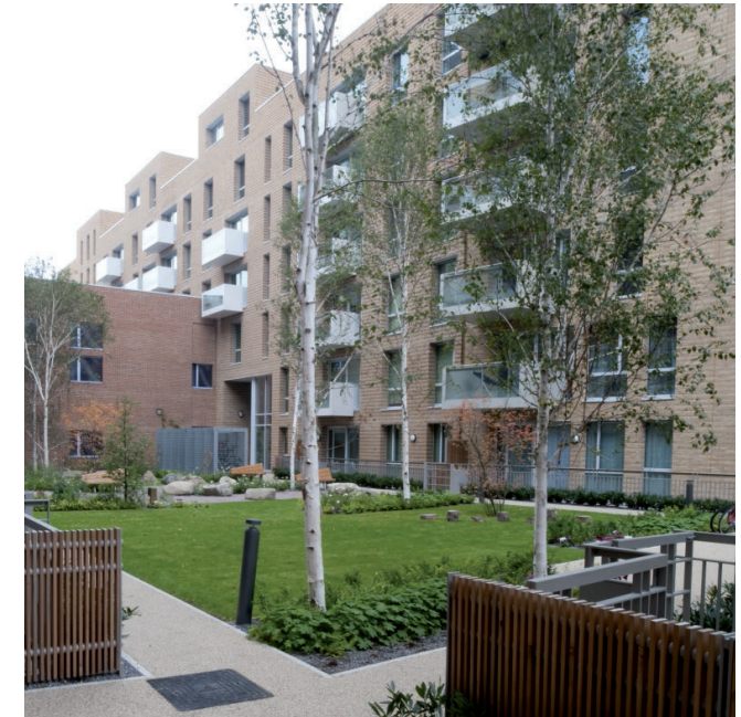
Figure 5.8: Photograph of a new housing development at St. Andrews, Bromley by Bow. Photograph by A&M Photography
