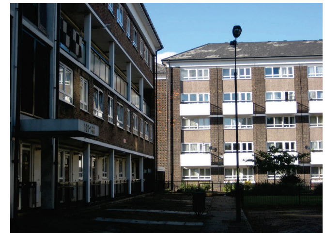
Figure 2.24: Photograph of a housing block within the Gibbs Green Estate
