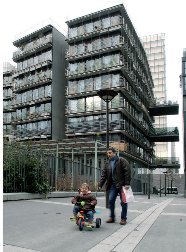
Figure 13.7: Photograph of a new housing development at River Gauche, Paris. Photograph by Urban Exposure
