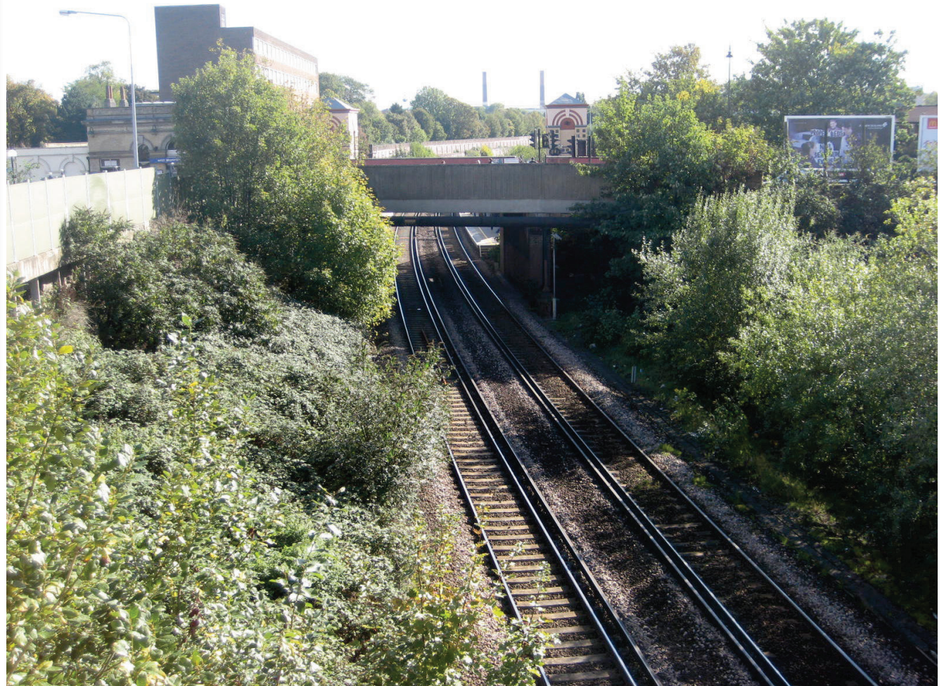
Figure 12.1: View looking south, along the railway line from EC2
