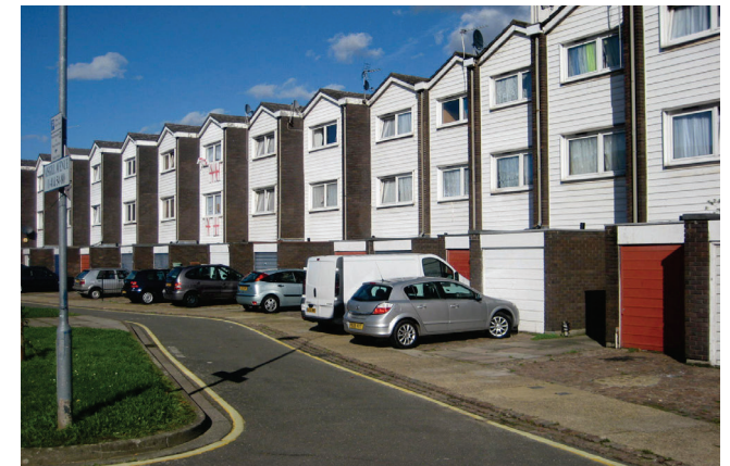
Figure 5.7: Housing within the West Kensington estate
